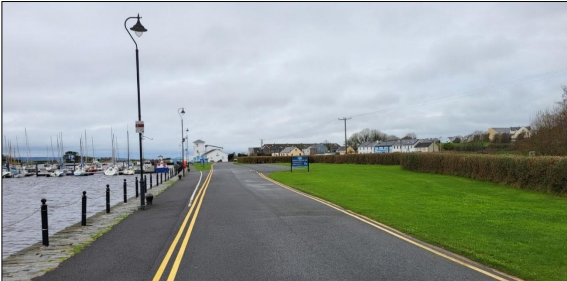
Plate 15-12 Looking west near Kilrush Marina with the site of the proposed trailhead carpark to the rear side of the hedge in the right of the foreground.
