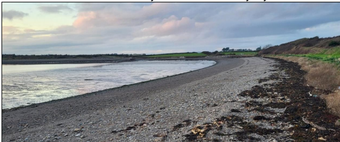
Plate 15-10 View from shingle shoreline at Brews Bridge beach looking west with the former railway line and site running along the grass embankment.
